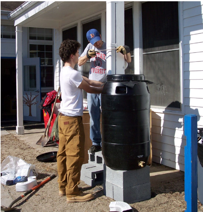
Installing a rain barrel (recycled pickled olive container)—photo by NLI
