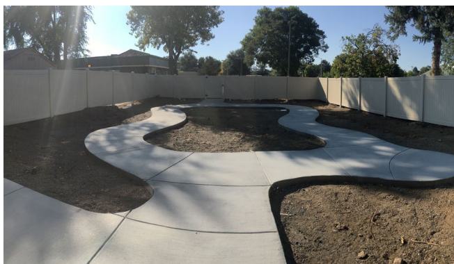
Concrete primary pathway.—photo by NWF
